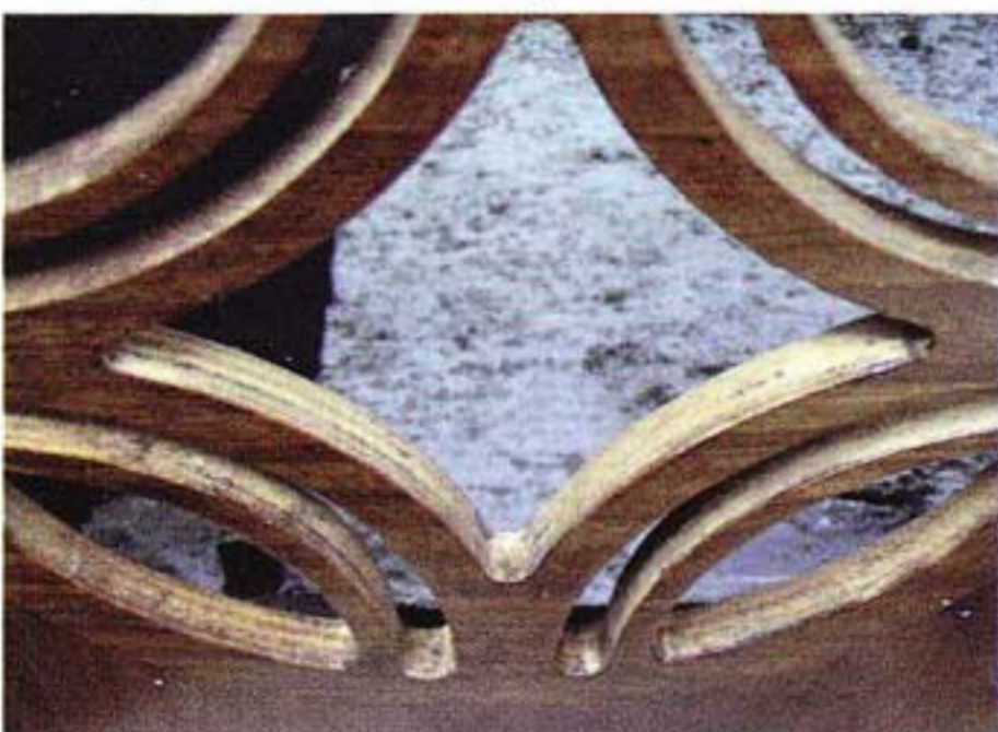
The fret end of the ply ready to paint
