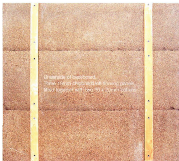
Fig 4: Underside of baseboard
